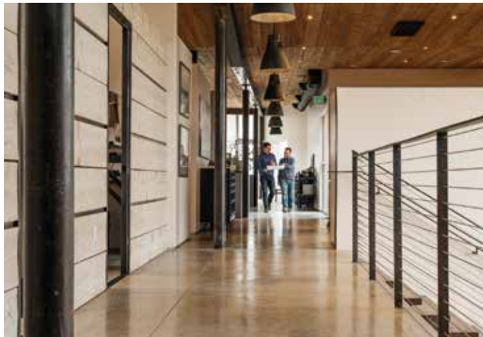
To add texture, Bowland used the rough-sawn floor joists over steel to side one wall of offices.
