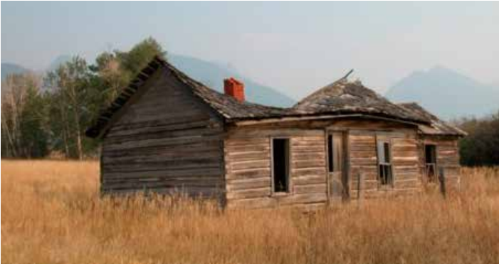
Before and after: The Indian Hills original homestead was so perfectly scaled and situated that Yellowstone Traditions suggested few changes except to make it last many generations as opposed to just one.
